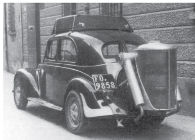
Wood gasifier-powered vehicle
