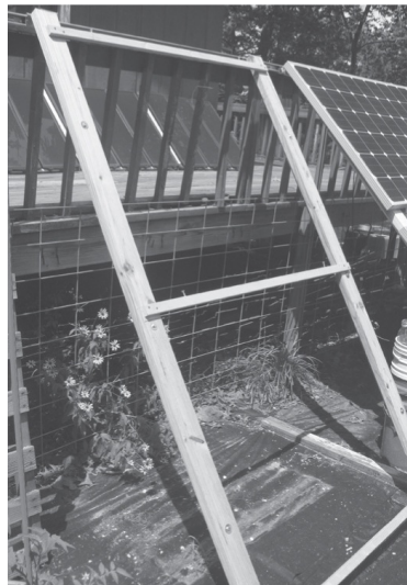
Wooden deck-mounted racking awaiting new panels
