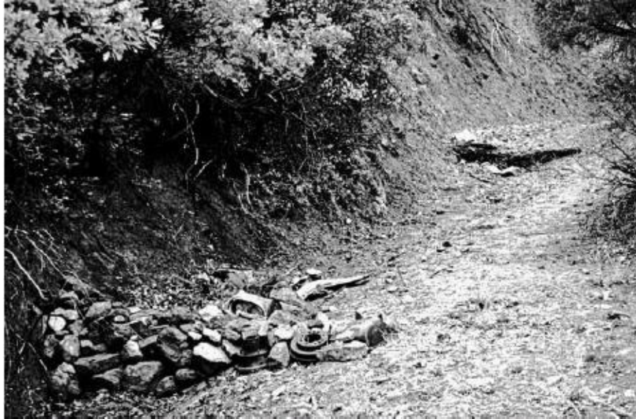
Two check dams will slow occasional stormwater in this Colorado mountain drainage, causing it to drop sediment and form terraces behind them. They were constructed of stones, brush bundles of Canada thistle (cut for weed control) and old car parts found nearby. [Credit: Peter Bane]
