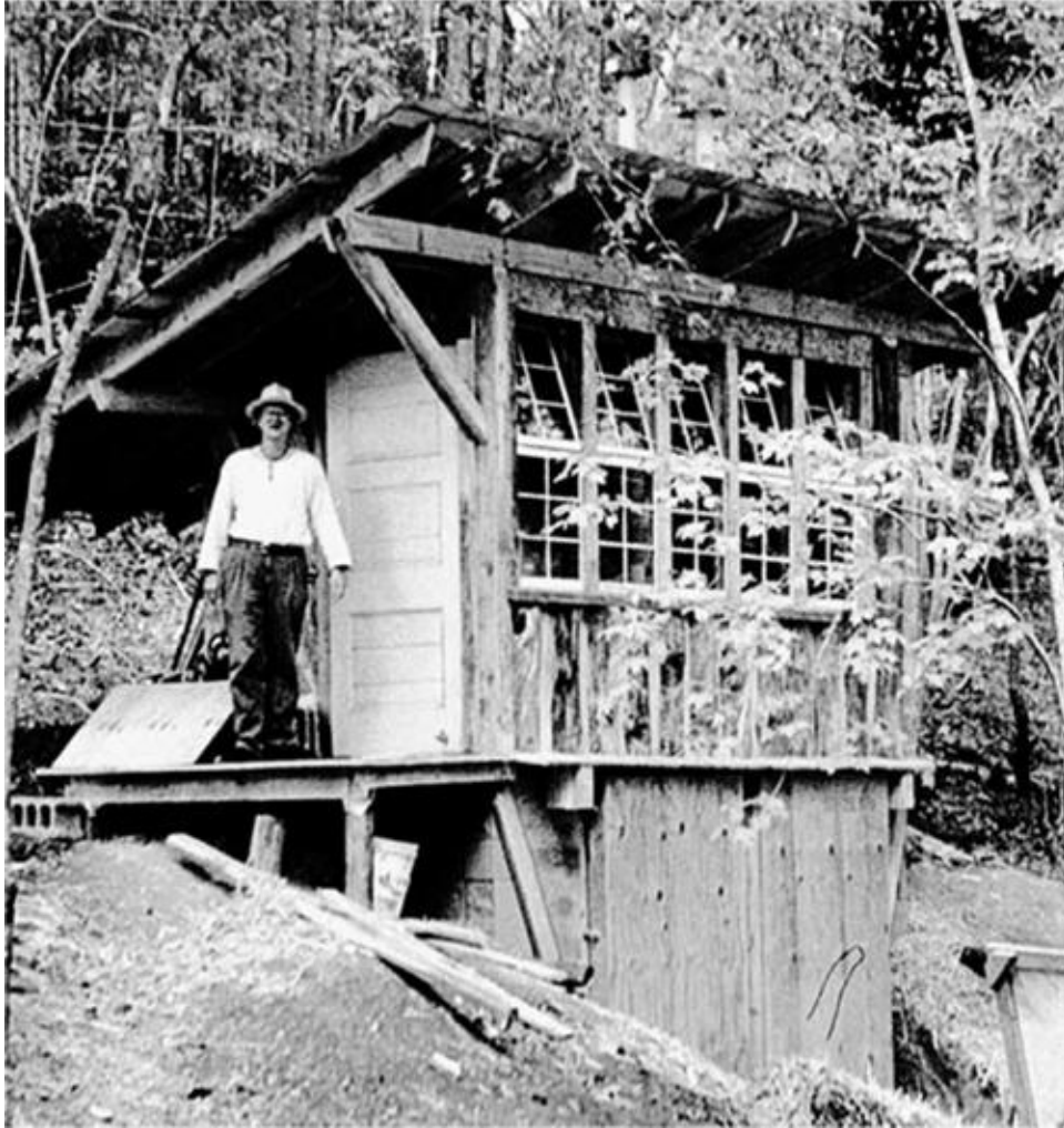
This free-standing mouldering toilet has two chambers built into a hillside. The south-facing glass front assists venting through the solar chimney. [Credit: Peter Bane]
