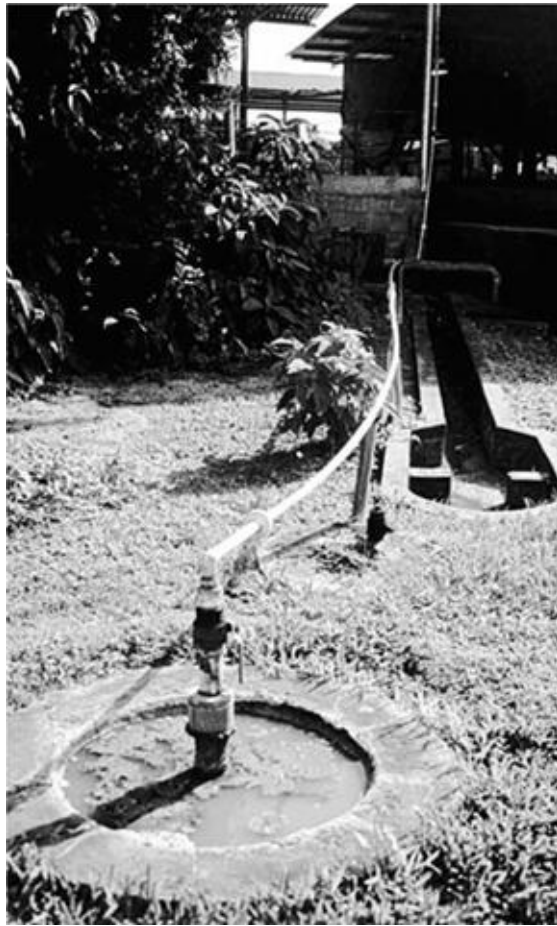
The above-ground portion of a digester that turns hog manure into methane and fertilizer. [Credit: Peter Bane]
