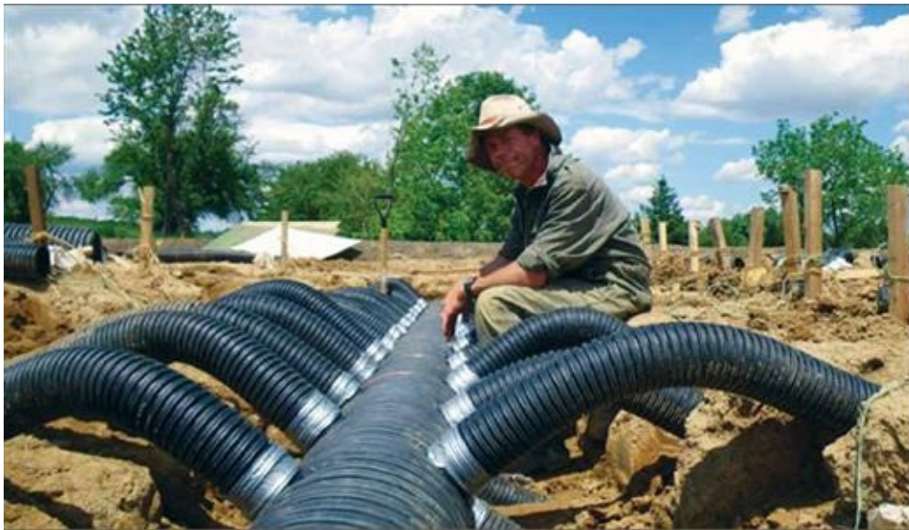
2. Installing the climate battery. [Credit: Ian Graham]
