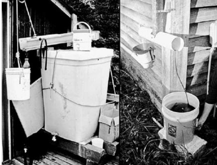
Pulley-and-pivot systems are one way to divert the first few gallons of dirty roofwater flushed by rain before directing runoff to storage. [Credit: Peter Bane]
