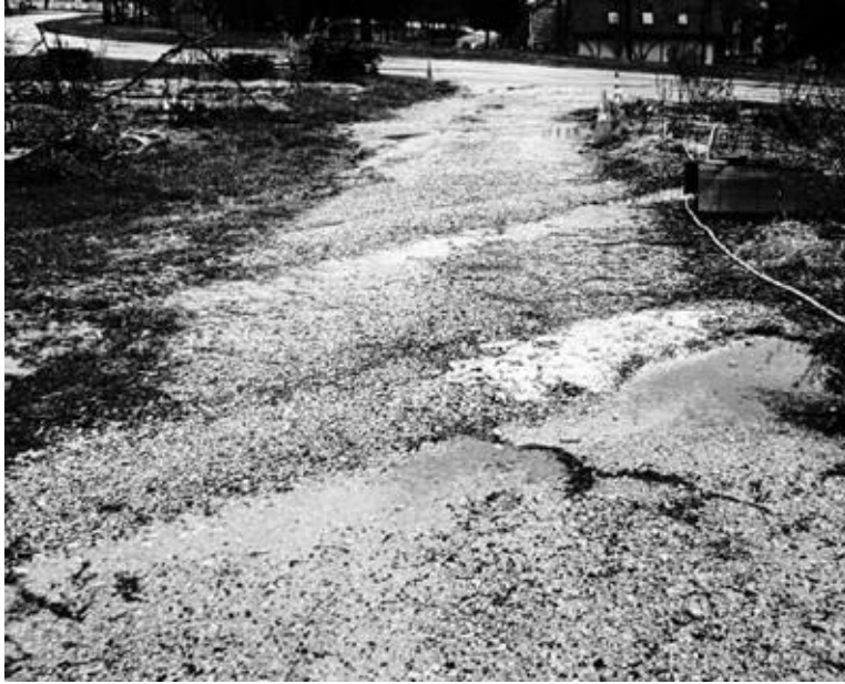
Water bars on the driveway divert surface runoff into garden swales while adding minerals to nearby soils. [Credit: Keith Johnson]
