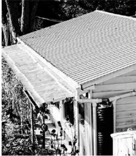
Enamelled metal panels form a durable roof with very high-quality runoff. [Credit: Creighton Hofeditz]
