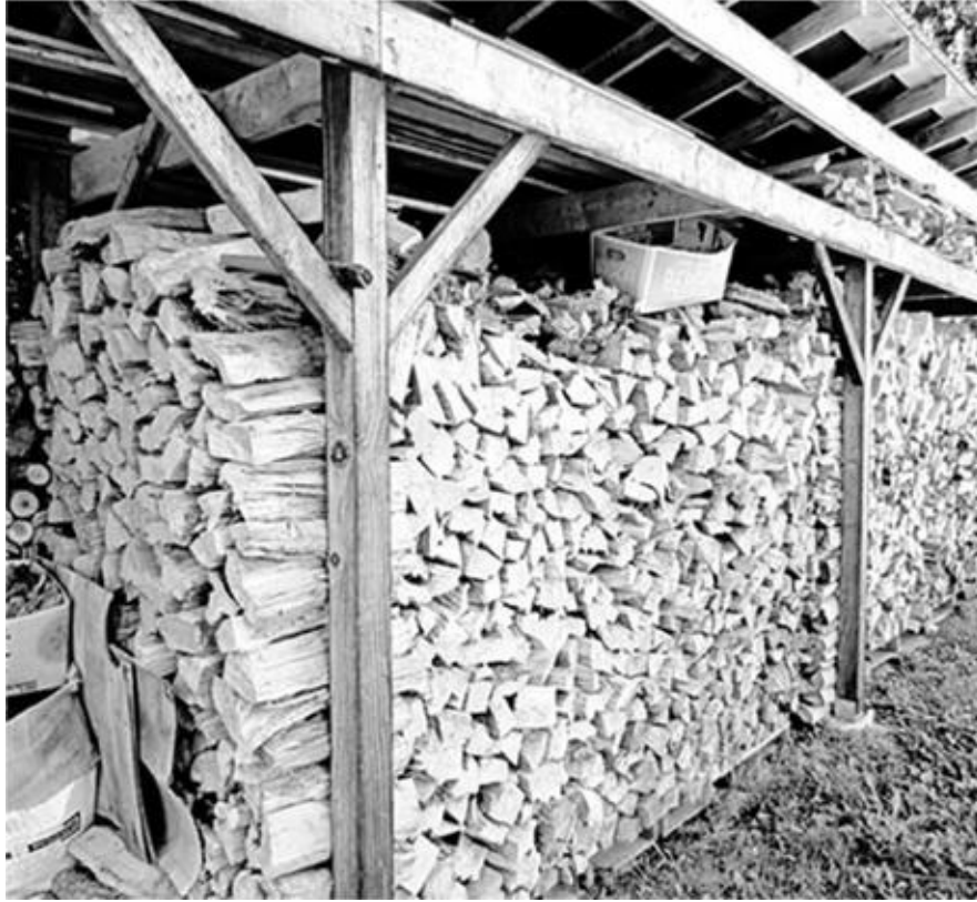
In this self-supporting design, longer logs are placed parallel to the length of the shed in between the posts to form “walls” between the bays. Then all other wood is stacked perpendicular to these walls. [Credit: Edward Carter]
