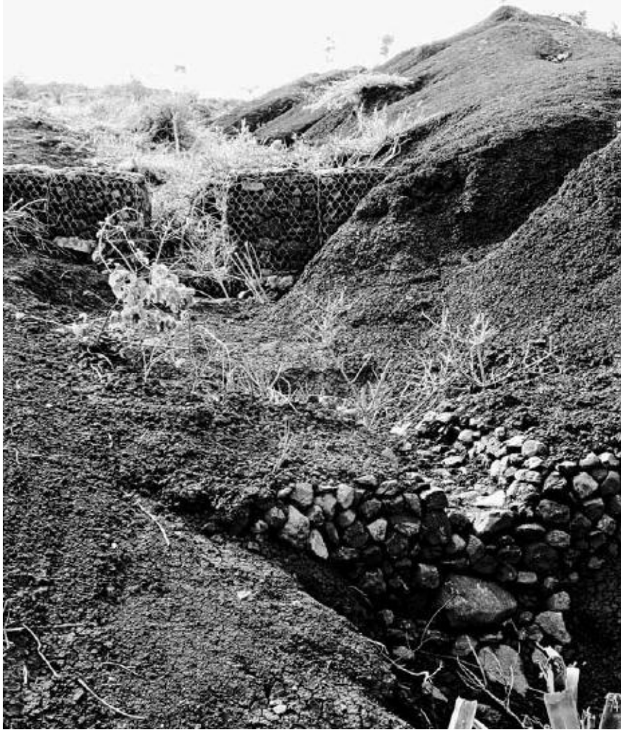
Two gabions above slow occasional heavy flows in this dry drainage while trapping sediments to repair a damaged watershed. The check dam downstream benefits from protection by the gabions; a partial terrace has already formed behind it. [Credit: treesftf via Flickr]
