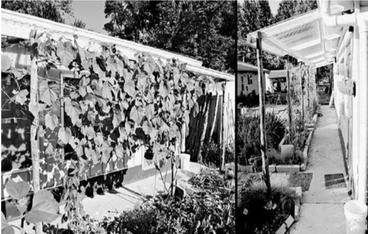
This grape-shaded awning integrates forces in conflict: seasonally variable sunlight, rain, foot traffic and entrance transitions. [Credit: Peter Bane]
