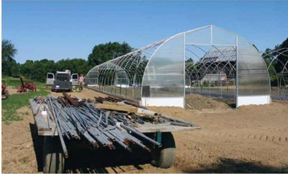
3. Erecting the greenhouse frames. [Credit: Keith Johnson]
