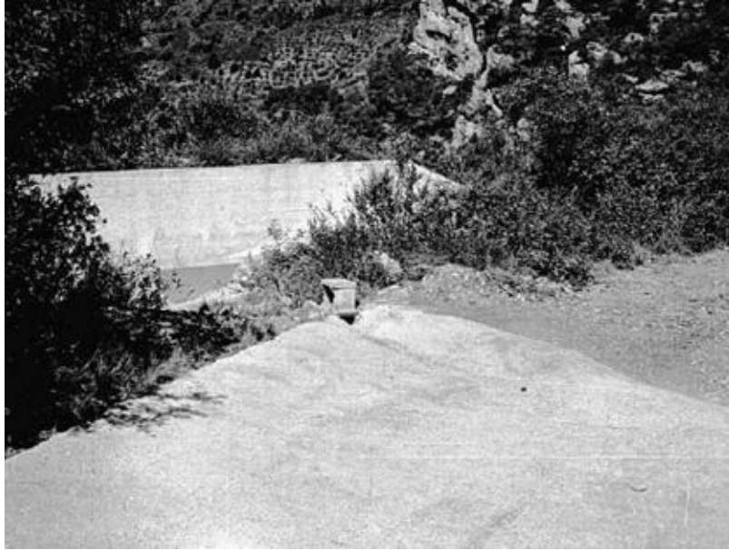
Runoff from roads and parking lots can be harvested for irrigation. This example in Catalonia drains to the open concrete tank visible behind the pavement. [Credit: Peter Bane]
