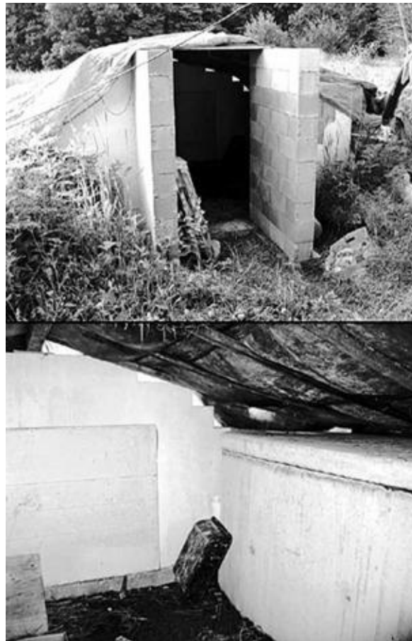
Entrance and interior of a root cellar built between two concrete water tanks made from precast septic vaults. (Design by Darren and Espri Bender-Beauregard) [Credit: Keith Johnson]
