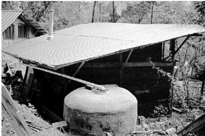
The simplest connection between a roof and a tank is a single pipe from a shed-style roof dropping directly into the cistern through a filter basket. [Credit: Peter Bane]
