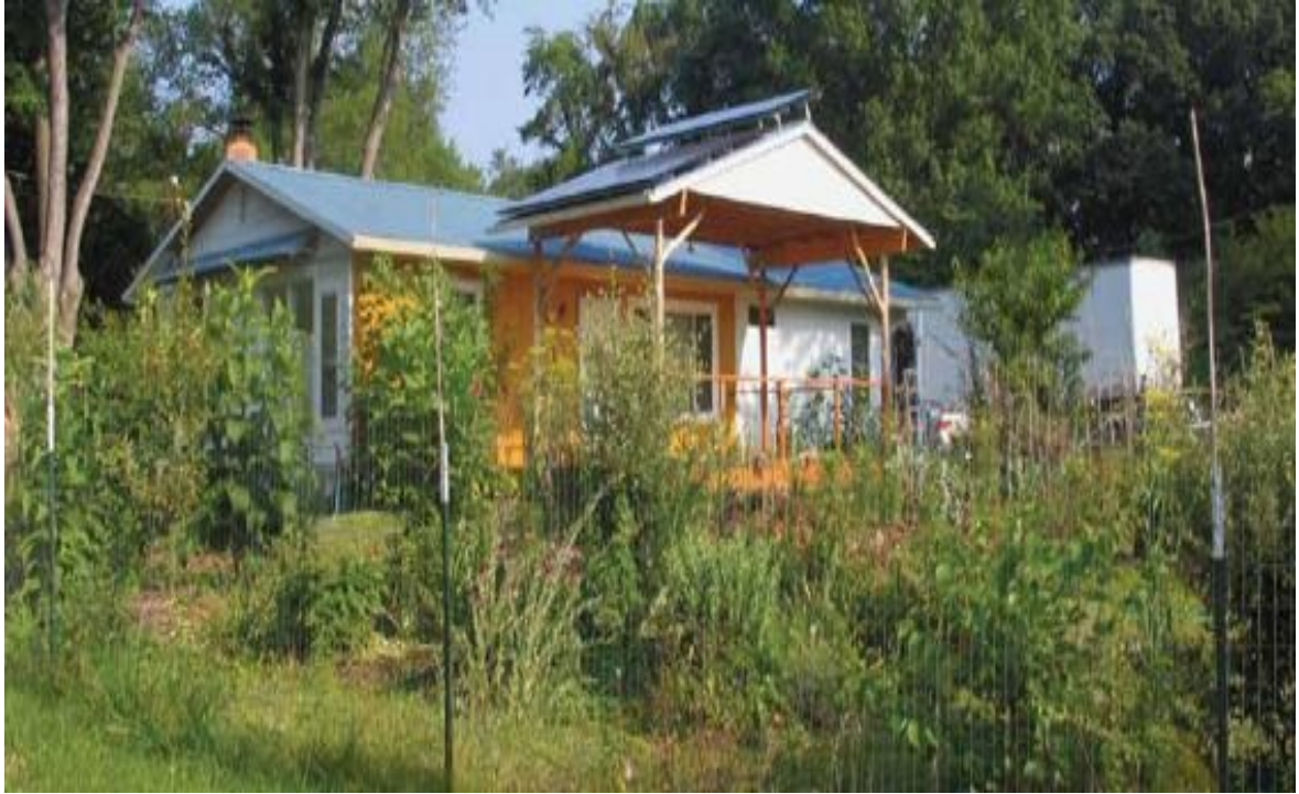
5. The summer following, photovoltaics were providing 100% of annual power use as the porch enhanced the utility of both house and garden. [Credit: Edward Carter]
