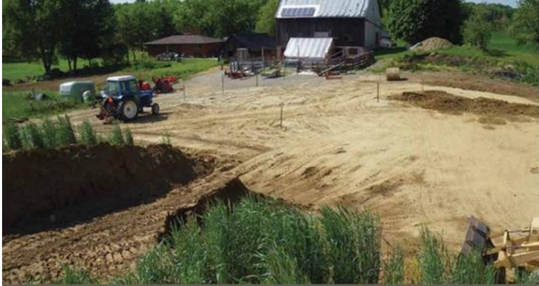
1. Preparing the site for two large greenhouses. [Credit: Ian Graham]
