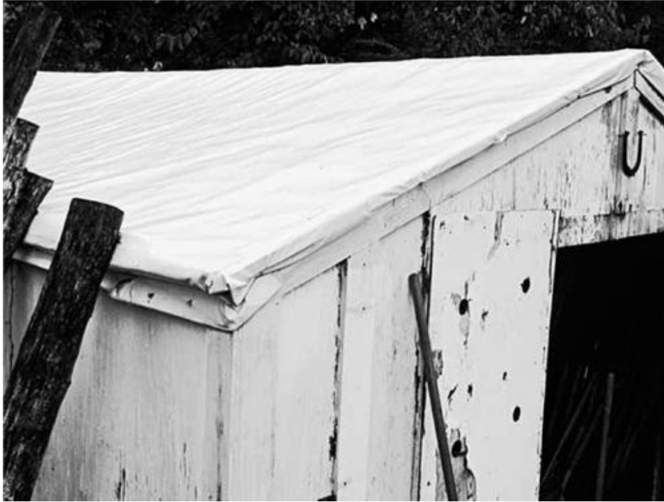
This ramshackle shed was given several years of new life by the addition of a $38 billboard tarp over a failing roof. [Credit: Creighton Hofeditz]
