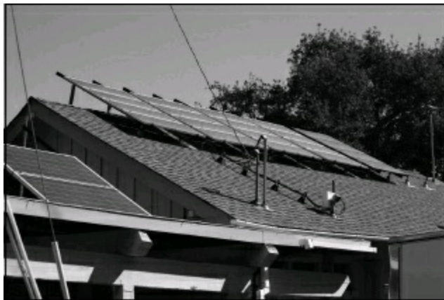
Small solar array powers entire house.
